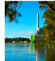
VALES POINT POWER STATION
